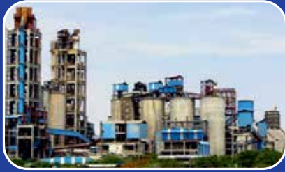
CEMENT PLANT MUKTYALA
