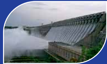
NAGARJUNA SAGAR DAM
