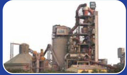
CEMENT PLANT MACHERLA
